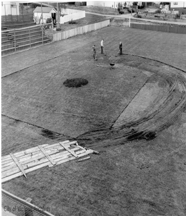
Construction of Jaycee National Little League in 1953
